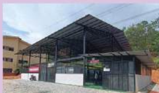
Well-equipped Electrical and Welding Workshops
